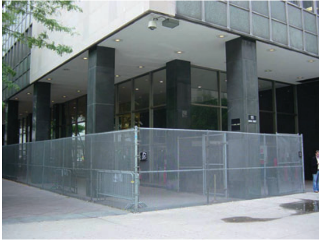
Figure 4 View looking northwest at a New York State office building located on Centre Street. The public plaza is closed to public access through the use of a ten feet tall wire mesh fence (photo by author)
